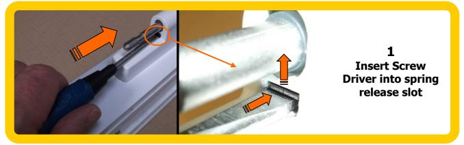
Insert a flat end screw driver into the slot found behind the pivot pin. The screw driver must be inserted under the leaf spring in order to lift the leaf spring up (i.e. away from the door frame)
