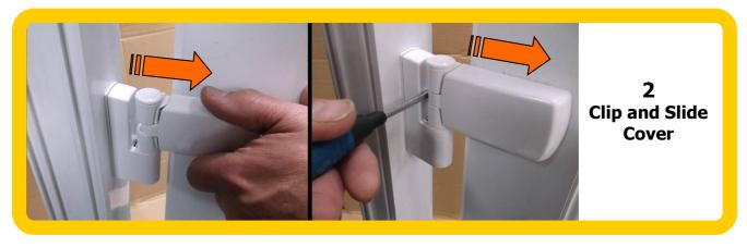
Pull the cover out towards the centre of the door. On release a click will be heard. If the cover does not open by hand a screw driver can be used behind the knuckle to gently assist opening. Repeat stages 1 and 2
