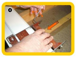
Adjust grip onto sash by sliding clamp block until it sits on inner edge of sash - Tighten with 5mm Allen key
