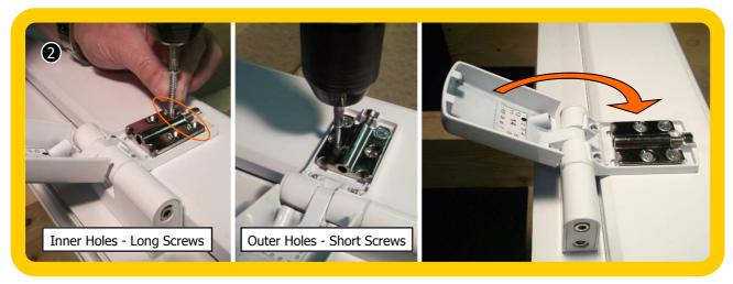
Secure Screw Plate with 2 x  $\emptyset$ 4.8mm screws in the inner holes ensuring they are the correct length to engage with reinforcing
